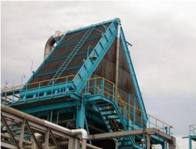
**Gambar 2.29** *Air Cooled Condenser*
