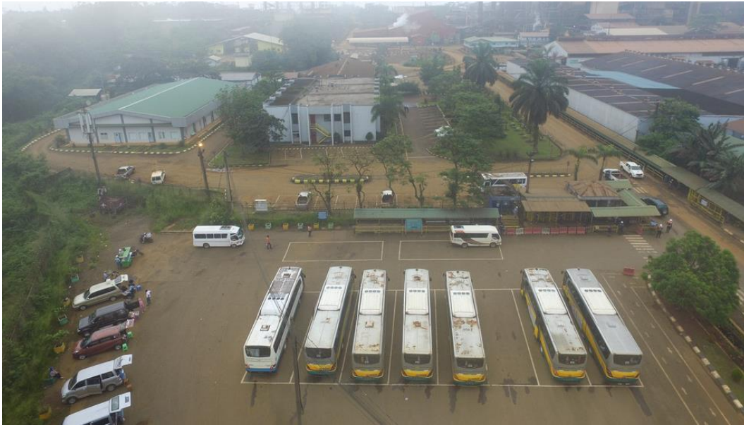
Gambar 4.33 Kondisi Gate 1 Plant Site
