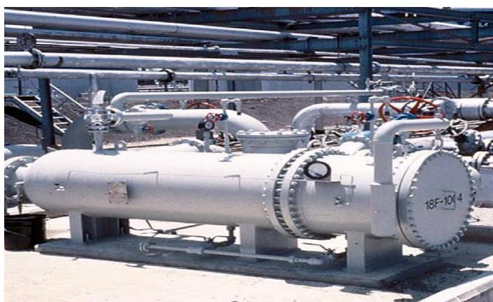
Gambar 3. 13 Instalasi *Filter Ultipleat High Flow* terpasang
