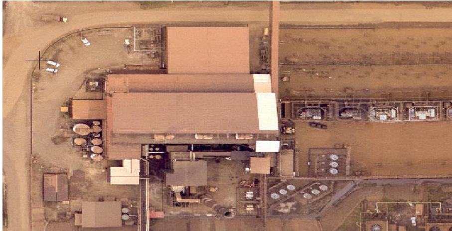
Gambar 3. 2 Lokasi Air dryer Hankinson PTVI
