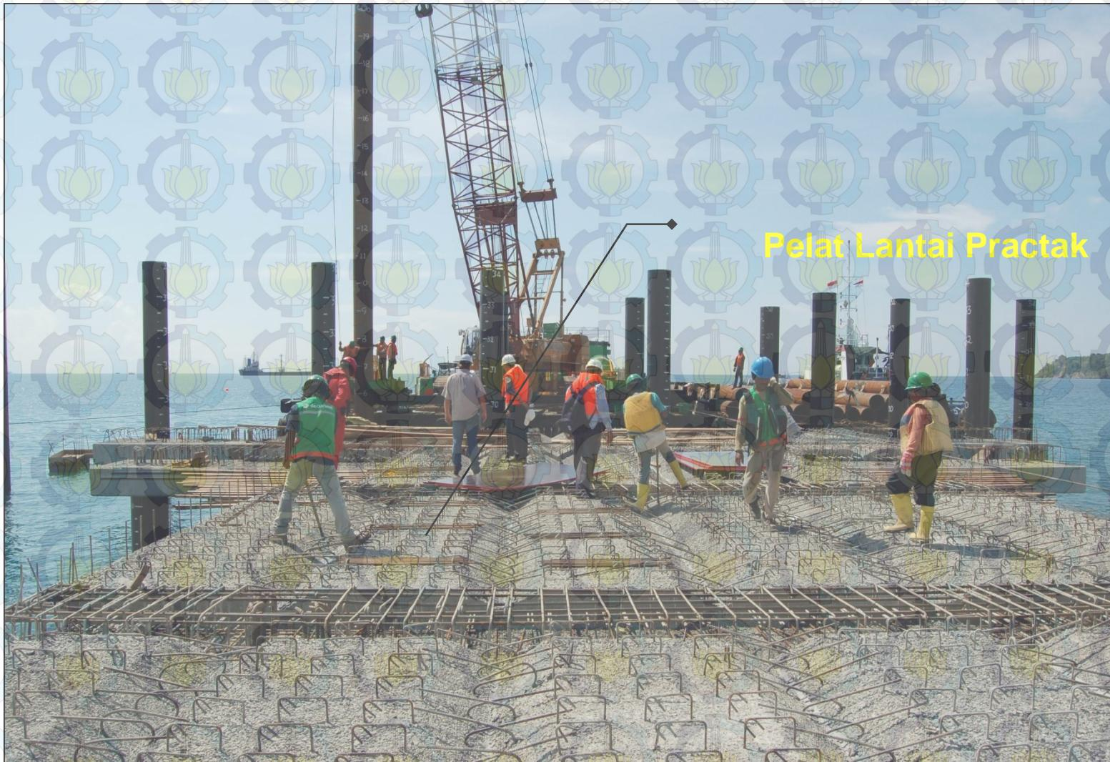
Sistem Pelat Lantai Half Slab Precast
