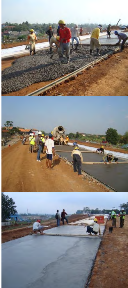
Gambar 4.22 Finishing Permukaan Beton
