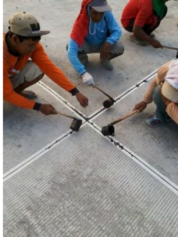
Gambar 4.34 Pengisian Joint Sealant
