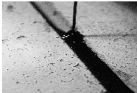
Gambar 2.9 Pengisian Joint Sealant
