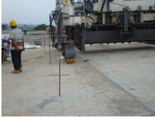
Gambar 4.26 Setting Concrete Paver
