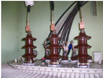
Gambar 2. 7 Bushing transformator
