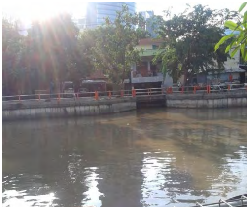
Gambar A.12 Kondisi Saluran Drainase ( Point Sources )
