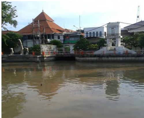
Gambar A.10 Kondisi Saluran Drainase ( Point Sources )
