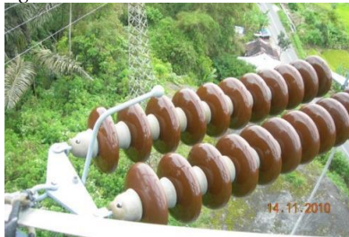
Gambar 3.7 Insulator tipe Horizontal string
