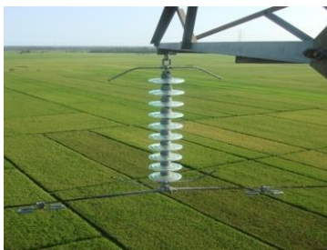
Gambar 3.8 Insulator tipe Single String
