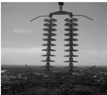
Gambar 3.9 Insulator tipe Double String
