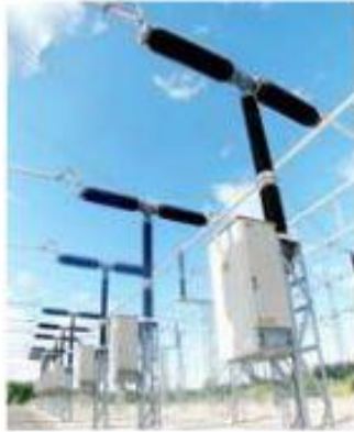
Gambar 2.4 SF 6 Circuit Breaker
