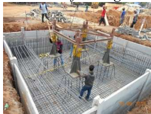
Gambar 4. 9 Penanaman fine angle dan base section
