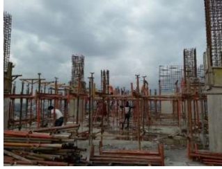
Gambar 4. 21 Perangkaian Scaffolding
