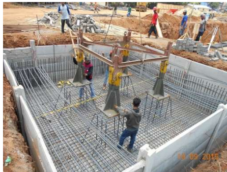
Gambar IV. 11: Contoh proses penanaman fine angle dan base section
