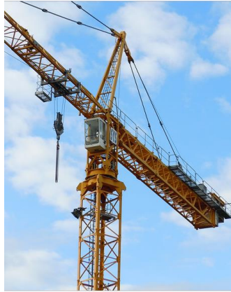
Gambar 2. 16 Tower Crane (Sumber: https://www.flickriver.com/photos )
