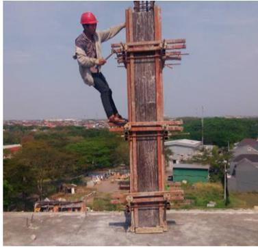
Gambar 5. 10 Tampak Bekisting Kolom
