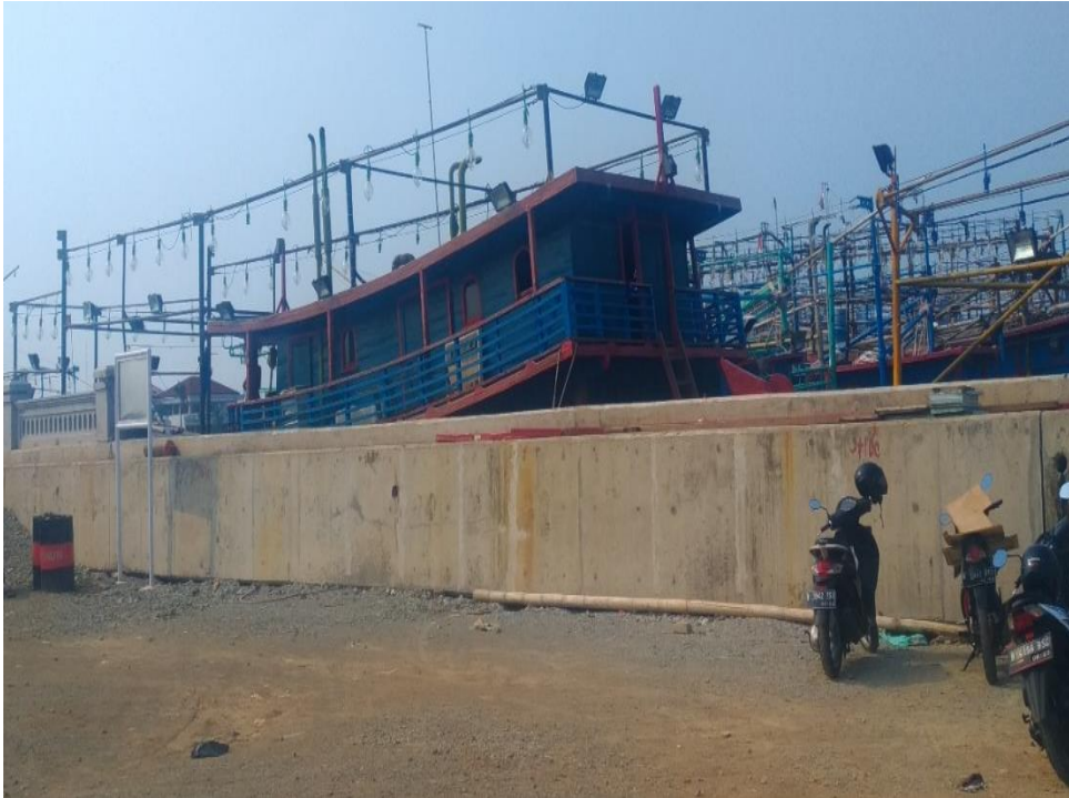
Gambar 4.2 Seawall NCICD fase A
