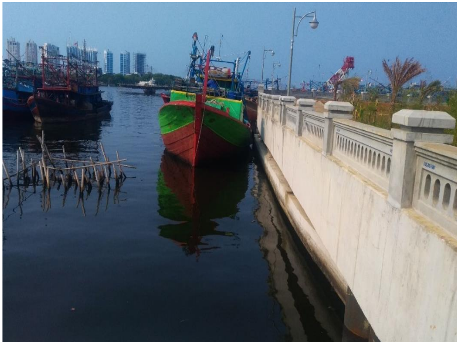
Gambar 4.3 Seawall NCICD fase A pluit
