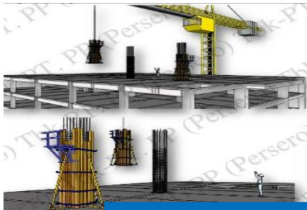
Gambar 4.12 Peningstalan bekisting kolom
