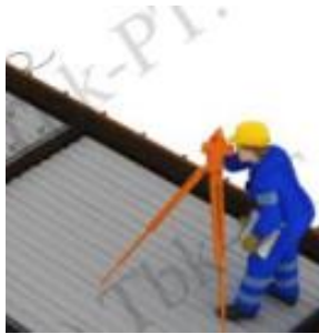
Gambar 4.10 Penentuan titik as kolom
