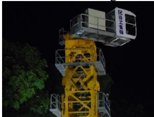
Sumber : PT. Brantas Abipraya Gambar 4.20 Pemasangan kabin diatas climbing crane
