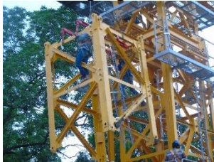
Sumber : PT. Brantas Abipraya Gambar 4.25 Peletakan mast section
