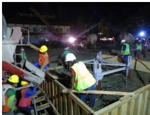
Gambar 4.17 Pengecoran pondasi tower crane
