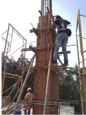
Sumber : PT. Brantas Abipraya Gambar 4.37 Pengecekan bekisting kolom
