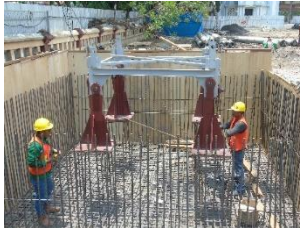
Gambar 4.16 Pemasangan fine angle tower crane
