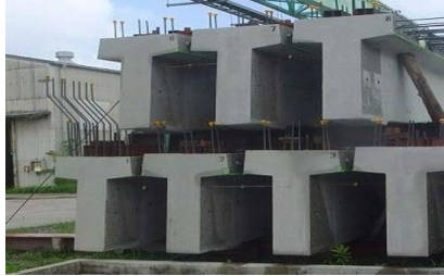
Gambar 2. 4 T Girder Sumber: Dokumentasi I&H Engineering
