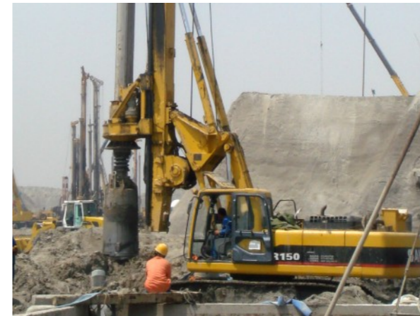
Zhengxi Railway passenger dedicated line project
