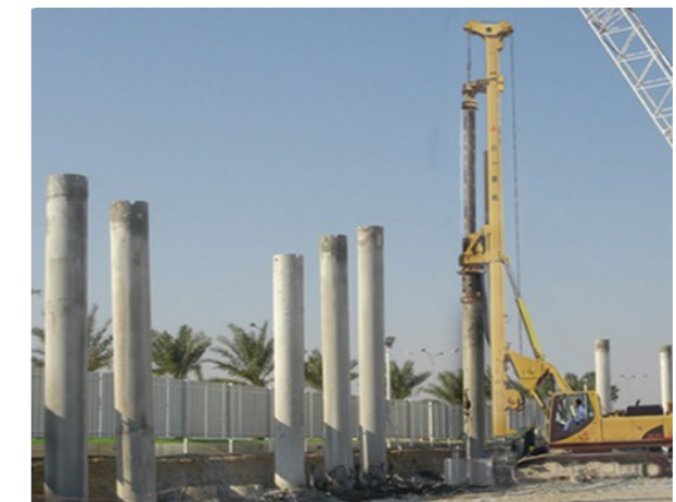
Airport construction in Doha, Qatar.
