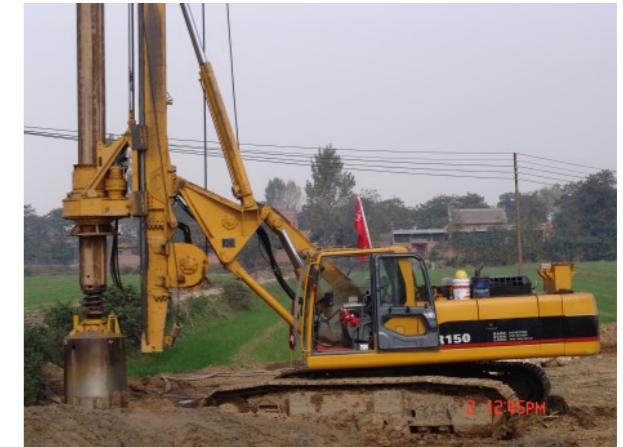
Wu Guang Railway construction site
