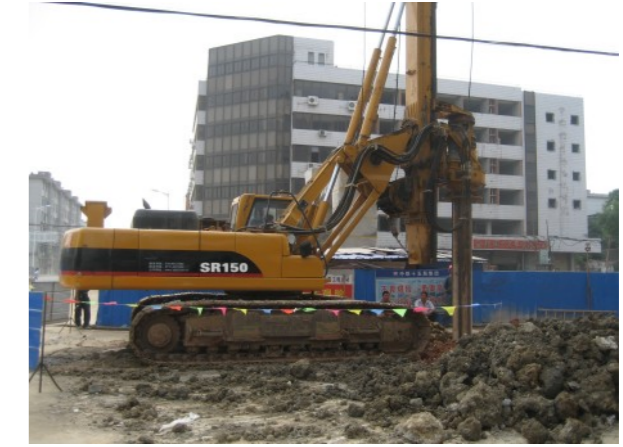
Hefei municipal construction site
