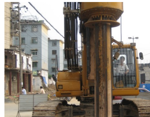
Xi'an urban construction site
