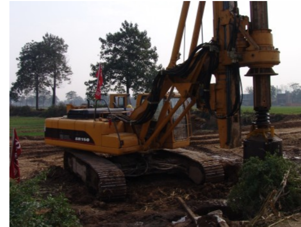
Yinchuan Yellow River Bridge construction project
