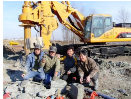
Efficient rock construction support
