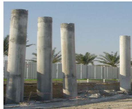
Soft overburden construction support
