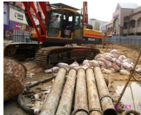
Small-diameter pile construction support
