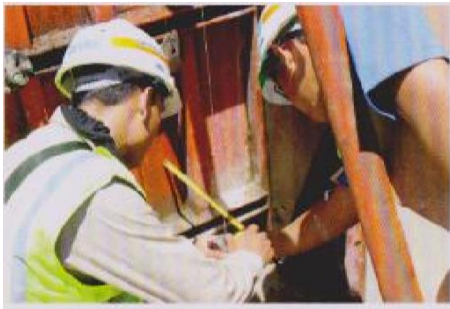
Gambar 5.5 : Pengecekan vertikal bekisting. Sumber : google image
