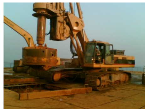
Over-water construction support
