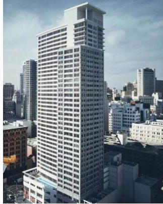
Gambar 2. 9 Gedung Paramount (Sumber: Henry, 2011)
