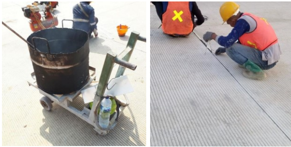
Gambar 4.37 Proses Joint Sealent
