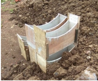
Gambar 4.12 Bottom Slab RCP Type A
