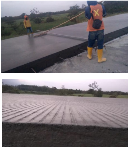
Gambar 4.34 Grooving Beton
