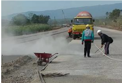
Gambar 4.28 Pembersihan Lean Concrete
