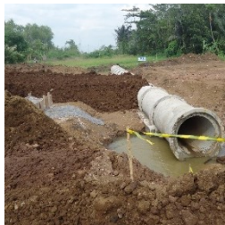
Gambar 4.13 Hampar Borrow Backfill
