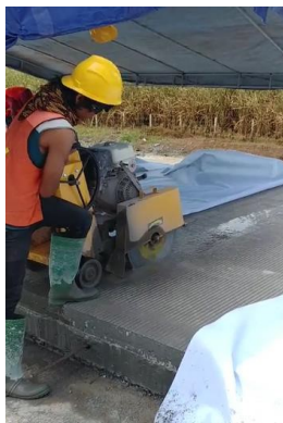
Gambar 4.36 Cutting Beton
