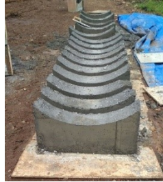
Gambar 4.12 Bottom Slab RCP Type A
