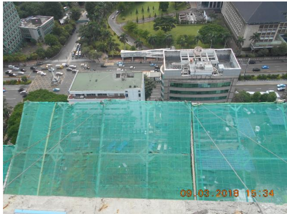
Gambar 2.5 Pemasangan Safety Deck
