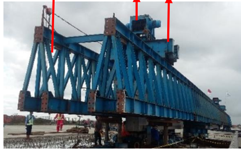
Gambar 4. 24 Bagian-Bagian Launcher Girder
