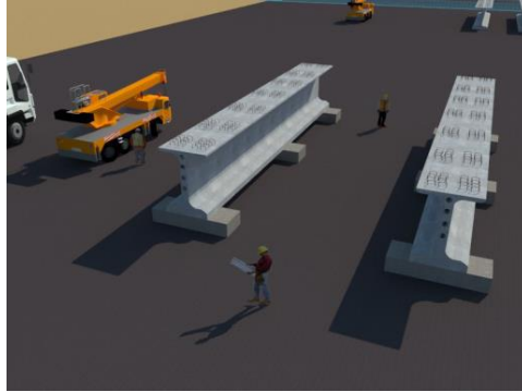
Gambar 4. 61 Proses levelling girder
