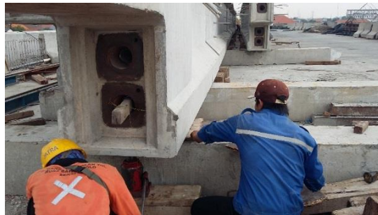
Gambar 4. 60 Setting Levelling Vertikal Balok
