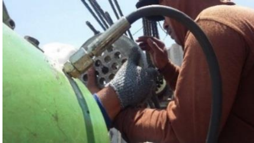
Gambar 4. 73 Proses Pemasangan Temporary Block
