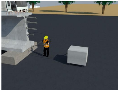
Gambar 4. 82 Proses Stressing Girder
