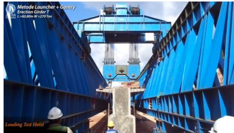
Sumber: PT. Jatra Sejahtera Gambar 4. 39 Loading Test Hoist
