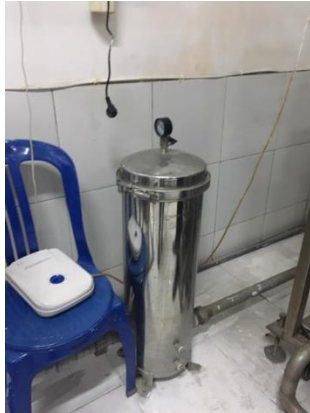
Gambar 4.2 Unit Cartridge Filter
