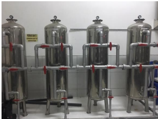
Gambar 4.1 Unit Rapid Sand Filter
