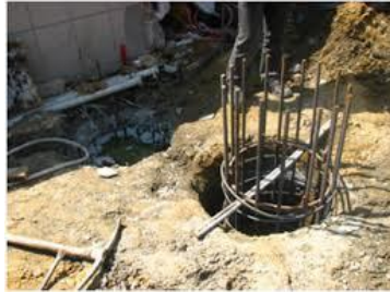
Gambar 4. 4 Pemasangan Tulangan Bore Pile (Sumber : http://www.jasaborpile.info/2016/04/pondasi-bore-pile.html )
