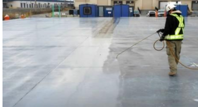
Gambar 4. 16 Curing Beton
