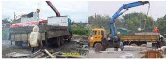
Gambar 6.7 Pengiriman Beton Precast
