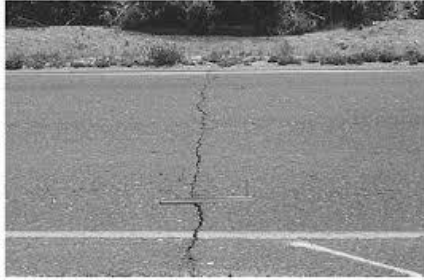
Gambar 2.7 Transverse Cracking
