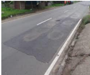
Gambar 2.10 Bituminous Patching
