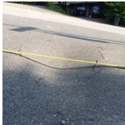
Gambar 2.4 Profile Distortion
