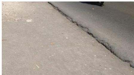
Gambar 2.9 Edge Deterioration
