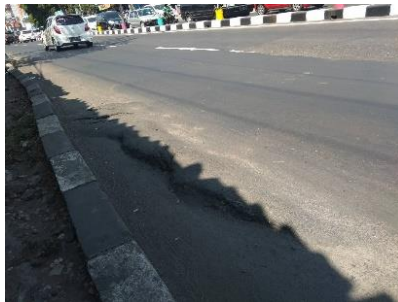
Gambar 2.8 Rutting (Alur)
