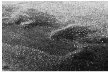
Gambar 2.4 Profile Distortion
