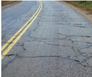
Gambar 2.5 Block Cracking
