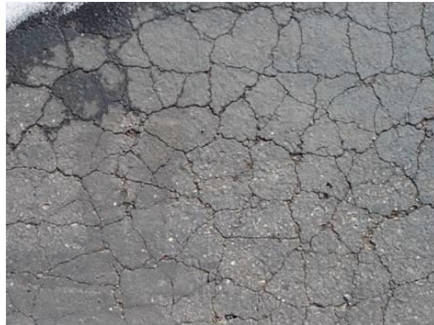
Gambar 2.2 Alligator Cracking
