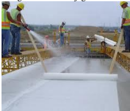
Gambar 5. 5. Curing Beton[13]
