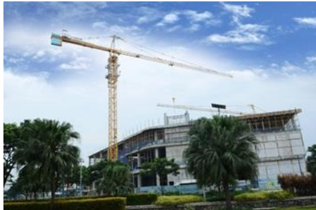
Gambar 2. 8. Tower Crane[9]
