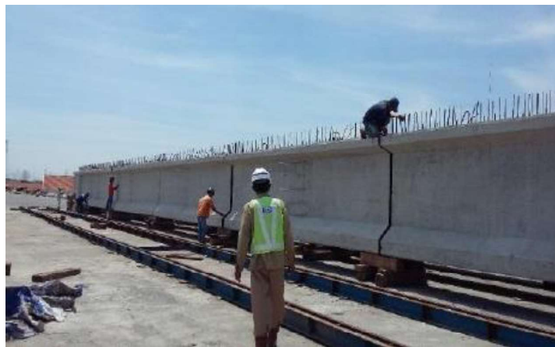
Gambar 4.30 Proses pengeleman
