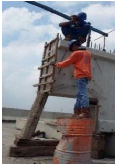
Gambar 4.34 Pemasangan bekisting patching
