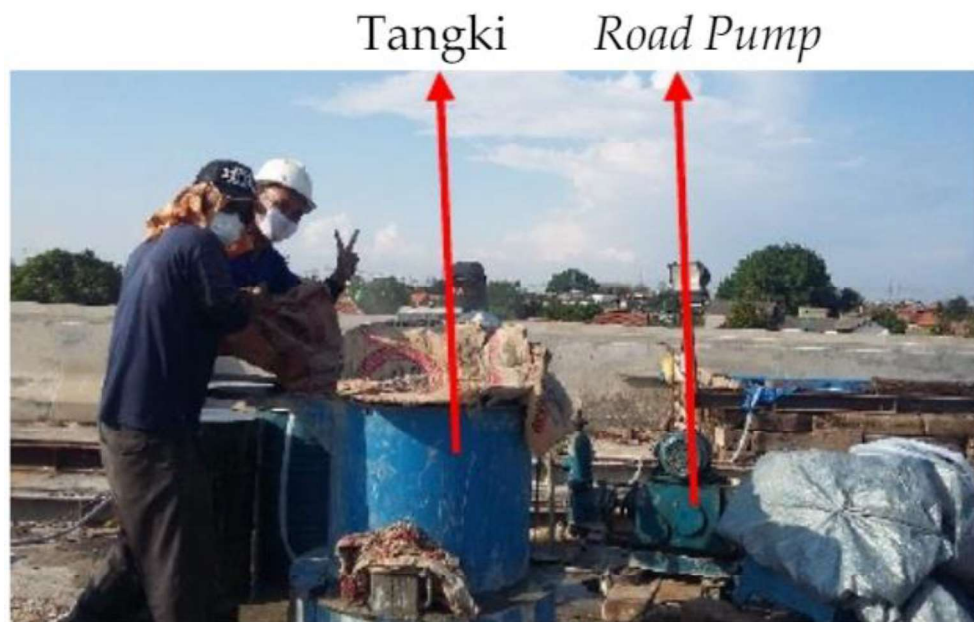
Gambar 4.36 Proses pencampuran material grouting
