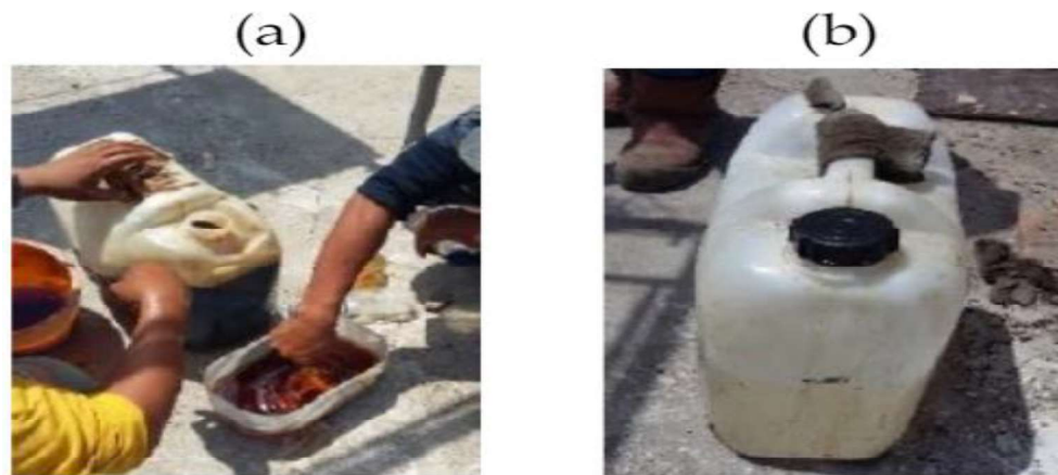
Gambar 4.29 Pencampuran lem beton (a) cardolit; (b) Epoxy
