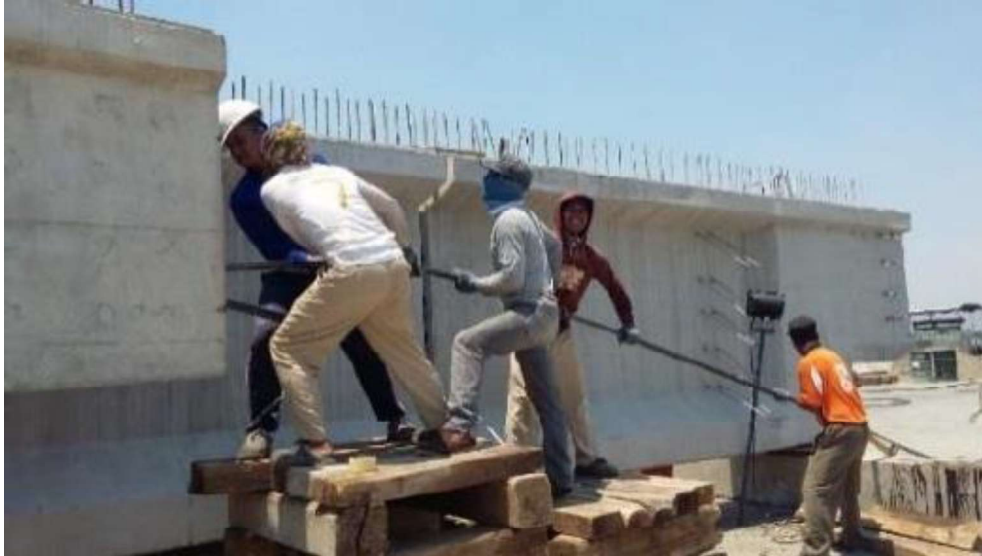
Gambar 4.20 Proses install strand
