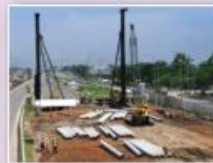
Piles Foundation for Bridges
