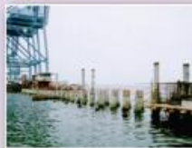
Piles for Marine Structure
