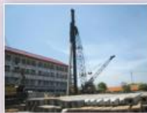
Piles Foundation for Building
