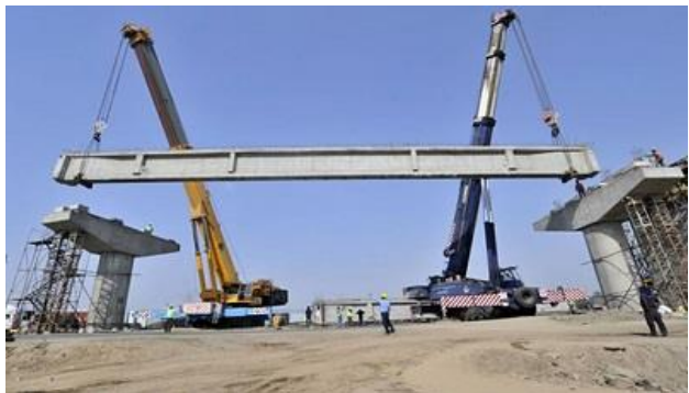
Gambar 2. 25 Ilustrasi Erection Girder (Sumber: www.testindo.com )
