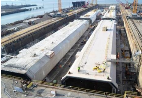
Gambar 5.25 Proses pabrikasi segmen immersed tunnel
