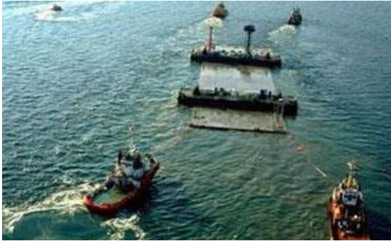
Gambar 5.28 Proses transportasi segmen
