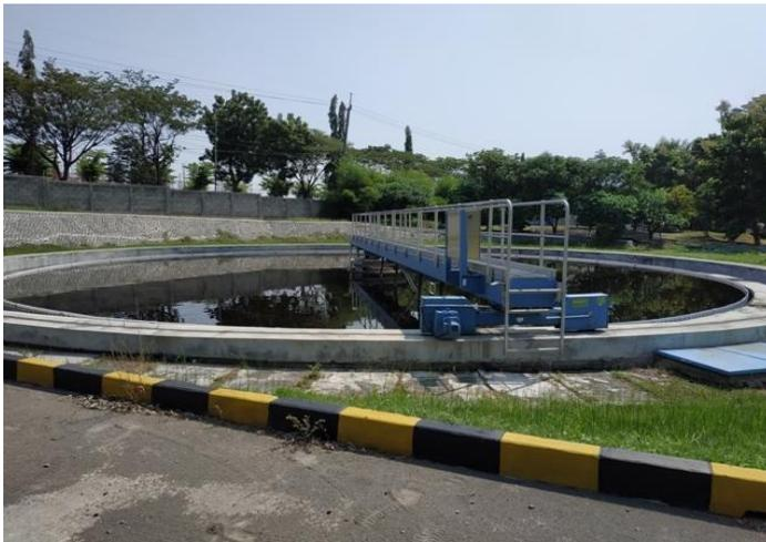
**Gambar 4. 5 Final settling tank**
