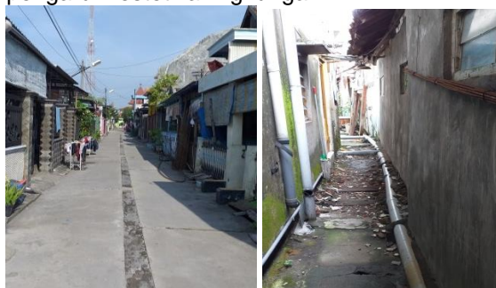
Gambar 4.26 Penanaman Pipa Utama SPAL
