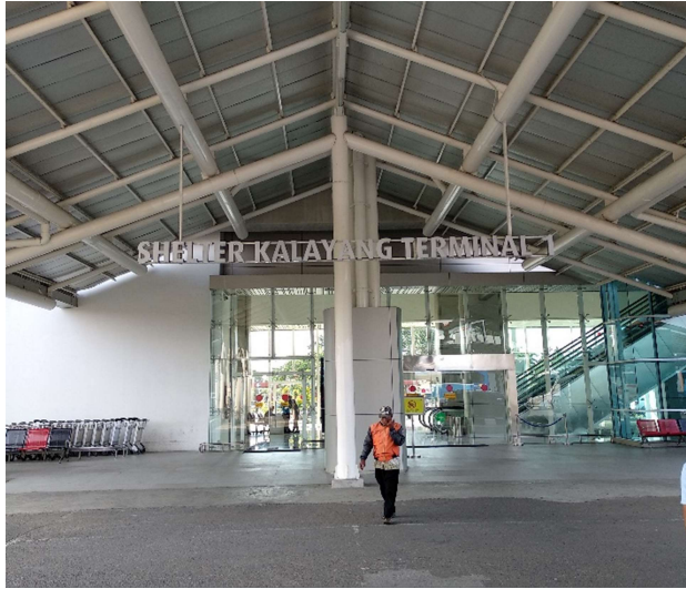
Gambar 4.15 Shelter Kalayang Terminal 1
