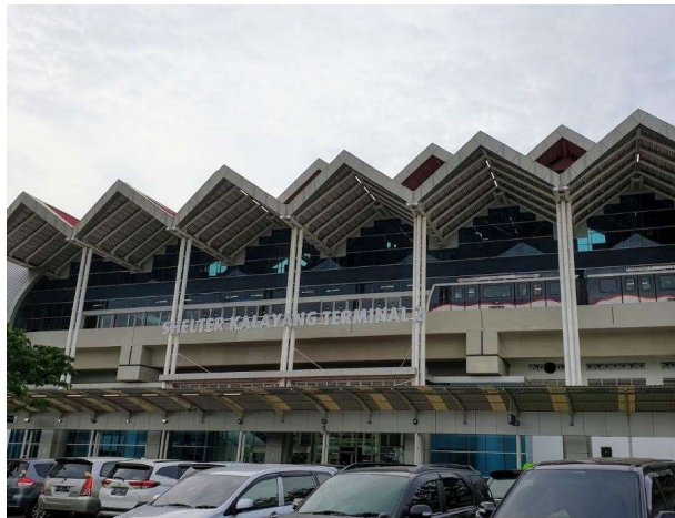
Gambar 4.16 Shelter Kalayang Terminal 2
