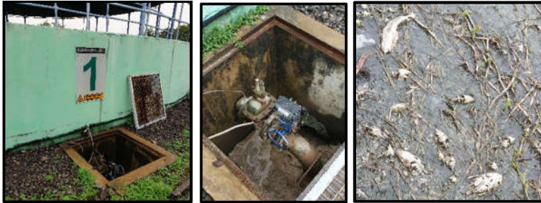
Gambar LC. 1 Kondisi Eksisting Pengelolaan Lumpur Alum PDAM (a) Unit Clearator (b) Saluran Drain Unit Clearator (c) Lumpur di Sludge Lagoon
