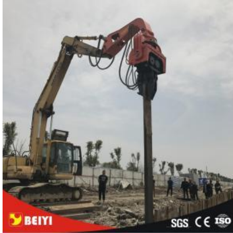
Gambar 2. 5. Vibratory pile driving (sumber: //google.com)
