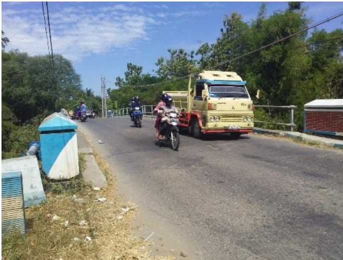
Gambar 1. 2 Jembatan Taap Existing
