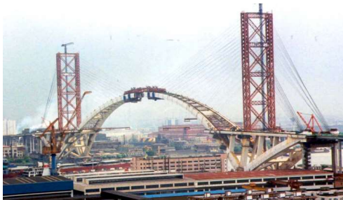
Gambar 3.7 Metode Balance Cantilever (Wong, 2012)
