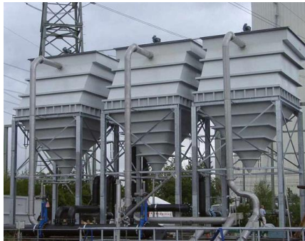
Gambar 2.2 Lamella Separator
