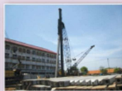
Piles Foundation for Building
