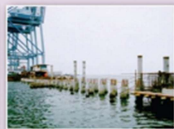
Piles for Marine Structure
