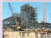
Piles foundation for Power Plant or Industrial Factory
