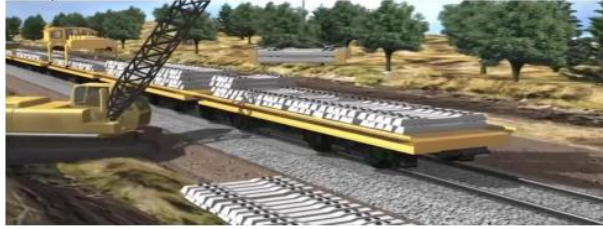
Gambar 5.36 menaikkan bantalan diatas Track Relaying Machine Sumber : Dirjen Perkeretaapian. 2017.
