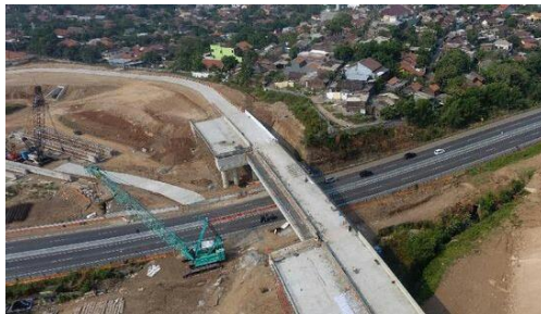
Gambar 1.4 Tampak Atas Jembatan Overpass STA 448+776
