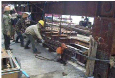
Gambar 7.3 Pemindahan Chain Block Formwork Traveller
