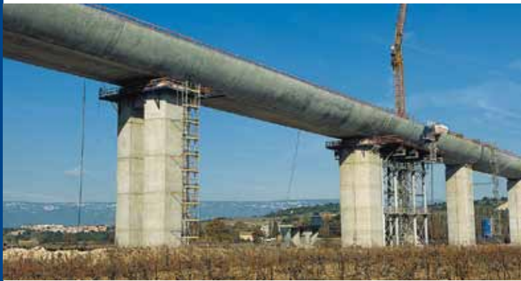
Vernègues viaduct, Mediterranean TGV line – France
