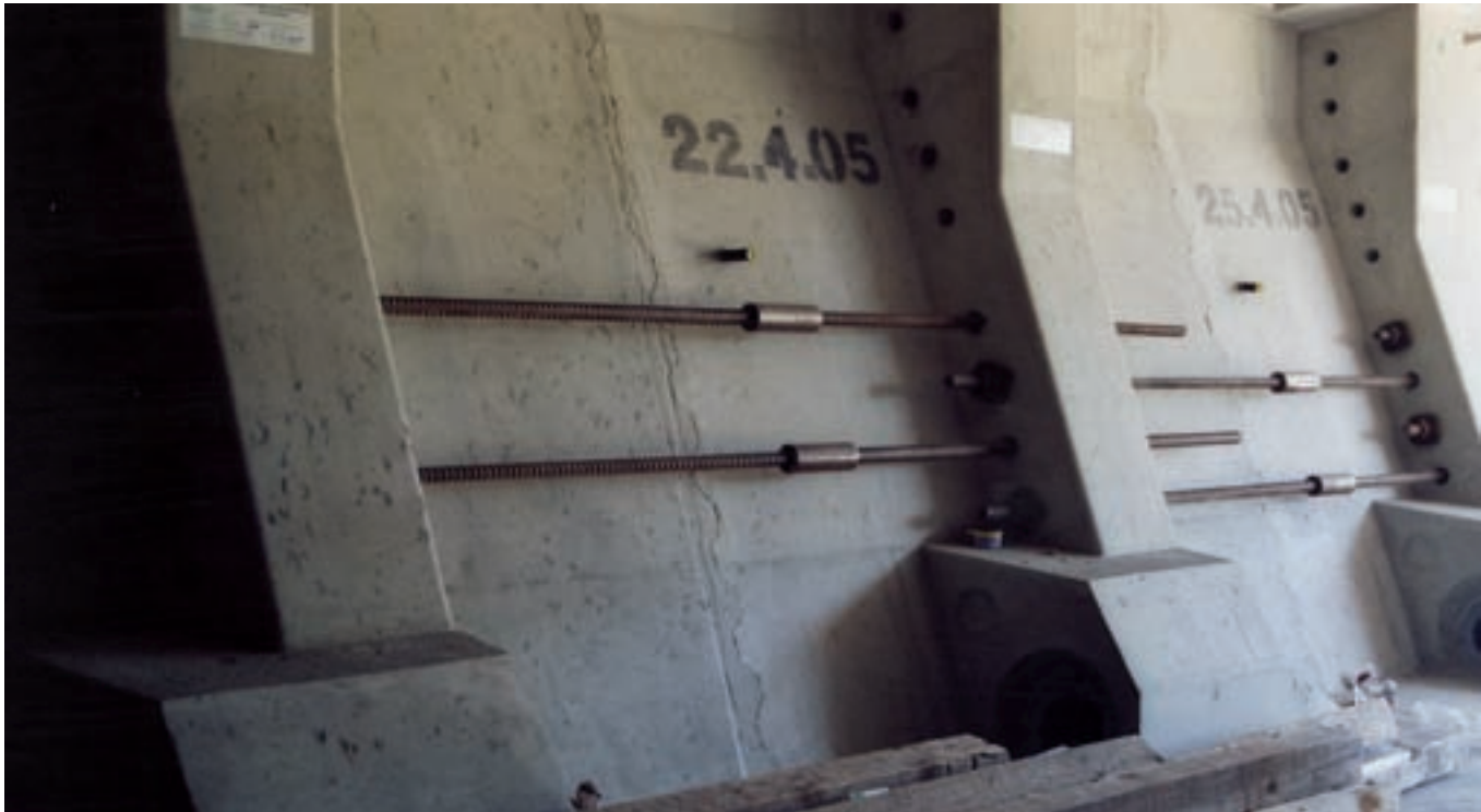
Typical Coupling, Uhlavu Bridge, Pilsen, Czech Republic
