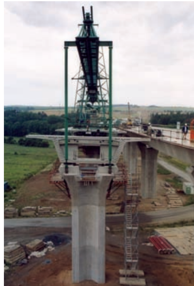
Uhlavu Bridge, Pilsen, Czech Republic
