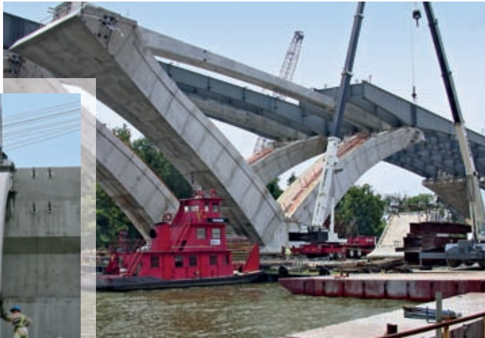
Woodrow Wilson Bridge, Washington, D.C., USA
