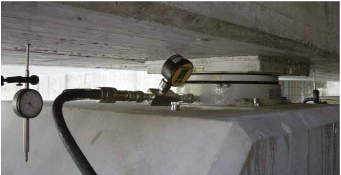
Weighable pot bearing Prébois viaduct – Switzerland
