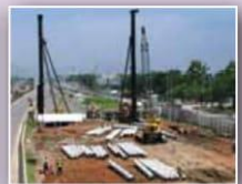
Piles Foundation for Bridges
