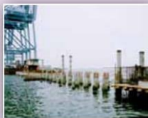
Piles for Marine Structure
