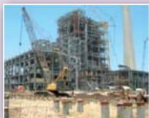
Piles foundation for Power Plant or Industrial Factory
