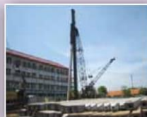
Piles Foundation for Building
