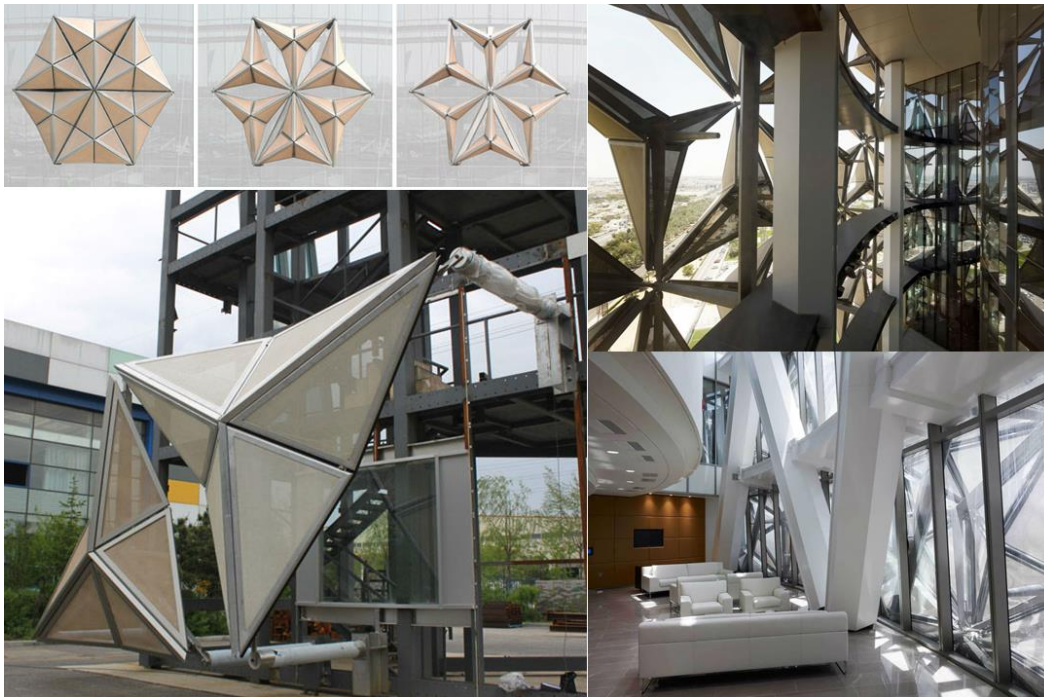
Gambar 2.49 Aktif shading device motif mashrabiya (Cilento, 2012)
