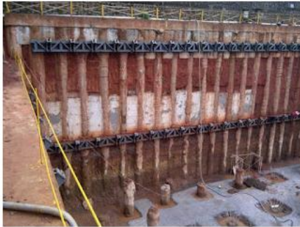
Gambar 2.17. DPT tipe Continguous pile (Sumber : Google Images)
