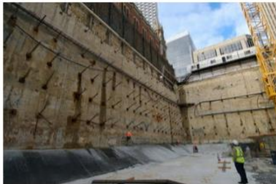
Gambar 2.16. DPT tipe diaphragm wall (Sumber : Google Images)
