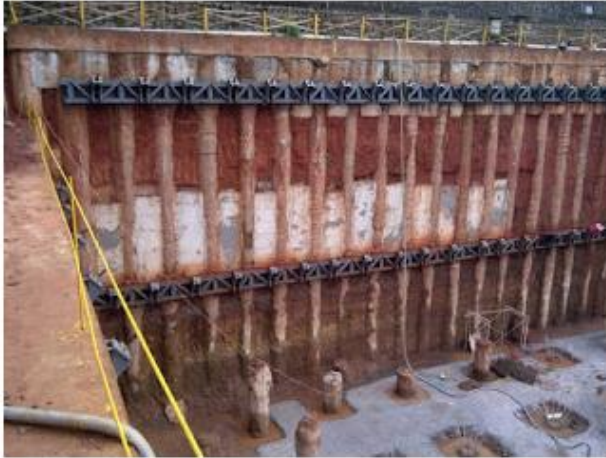
Gambar 2.17. DPT tipe Continguous pile (Sumber : Google Images)
