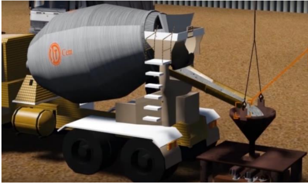
Gambar 6.14. Proses Pengecoran Kingpost Sumber : Google Images
