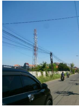
Gambar 4. 22 Jaringan Telepon (BTS)
