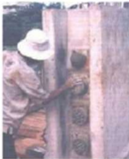
Gambar 2.19 Proses grouting dan patching
